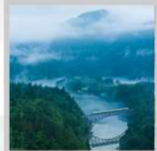
"TADAMI FIRST BRIDGE"
